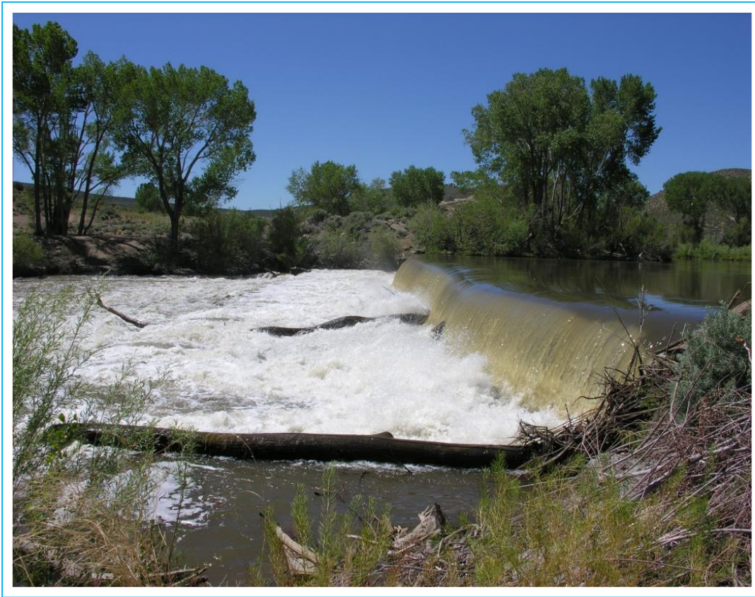
Photo 17. Historic Mexican Dam
