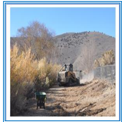
Mastication fuels treatment along the Mexican Ditch Trail
